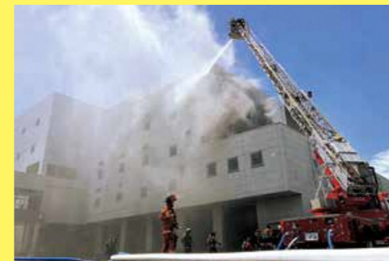
Fire at the Environmental Center (May 2023)
